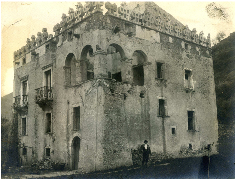
The front and side view (west-south) of the tower.
